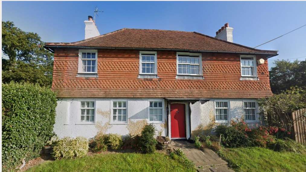
Image capture: July 2022 © 2023 Google. Above: View of Cooper Cottage from the A272.
